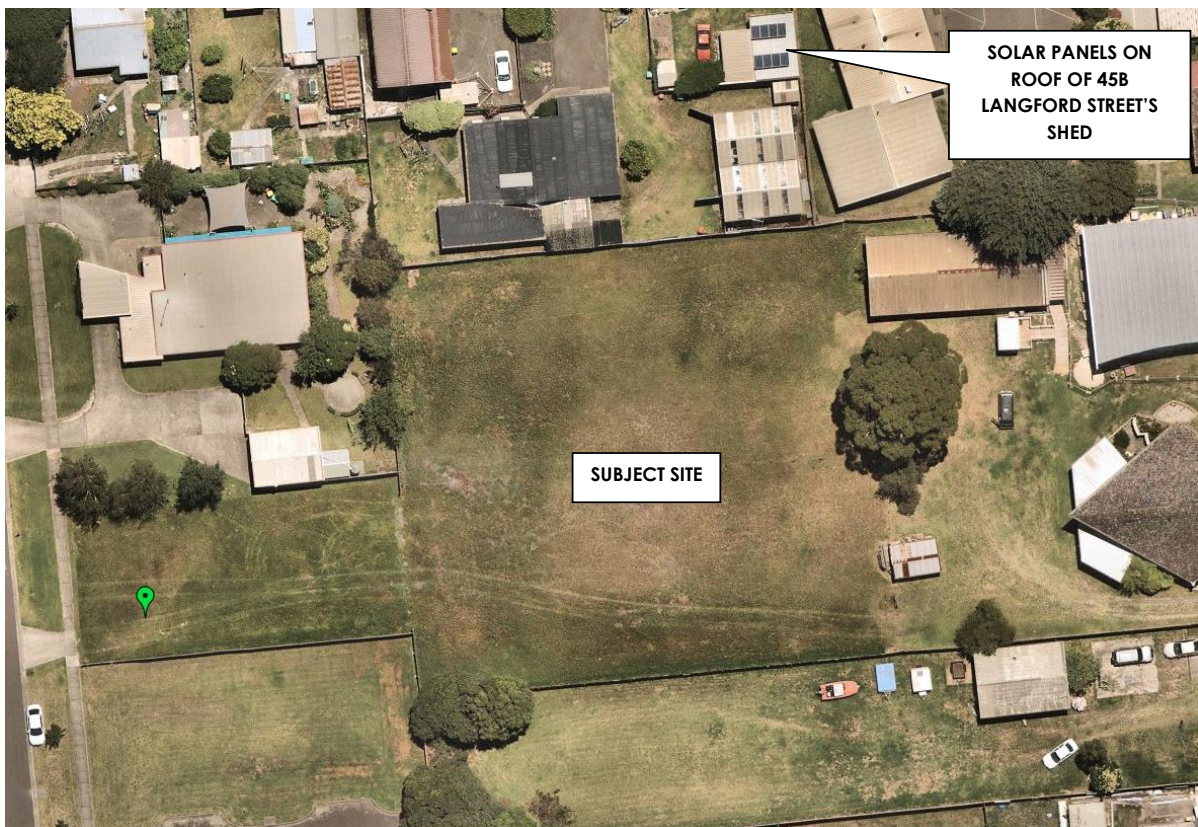
Figure 14: Location of Rooftop Solar Energy Facilities adjoining 5 Parer Avenue (photo source: Nearmap, January 2021)
