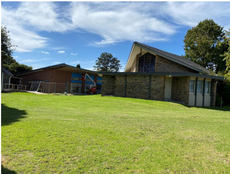
Photograph 15 – Rear view of the St. Andrew's Presbyterian Church site at 34 Fowler Street, facing east from the rear boundary shared with the subject land
