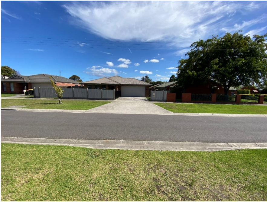
Photograph 20 – View of the existing dwelling at 8 Parer Avenue opposite the subject site
