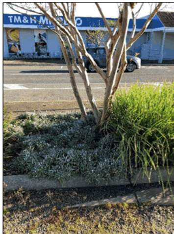
Figure 2.16. Base of tree 1 with existing concrete curb
