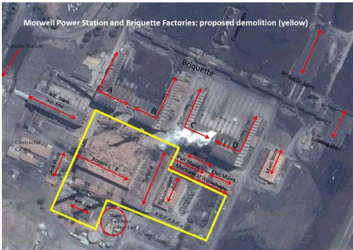
Fig 1: Aerial showing area to be demolished
