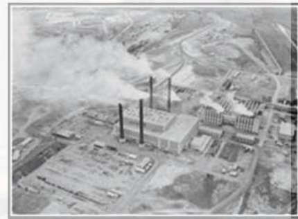
Industrial - Power - The combined brown coal electricity and briquette undertaking of the State Electricity Commission, at Morwell, Victoria, 1961 National Archives of Australia
