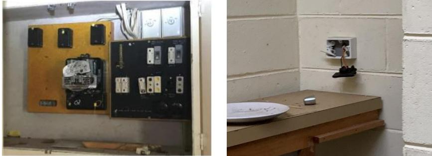
**Figure 4 Pavilion Meter Box and Damaged Power Point**
