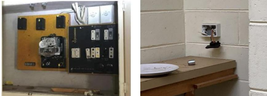
**Figure 5 Pavilion Meter Box and Damaged Power Point**
