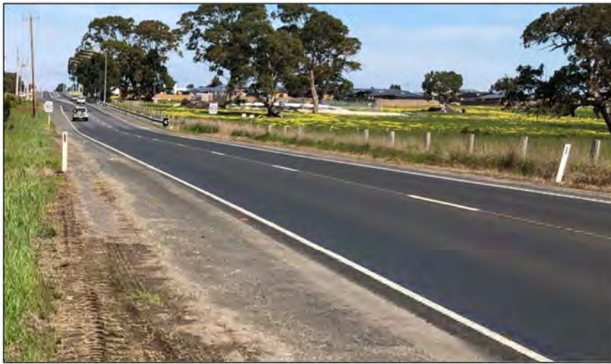
FIGURE 5: TRARALGON-MAFFRA ROAD FACING SOUTH (SUBJECT SITE ON RIGHT)
