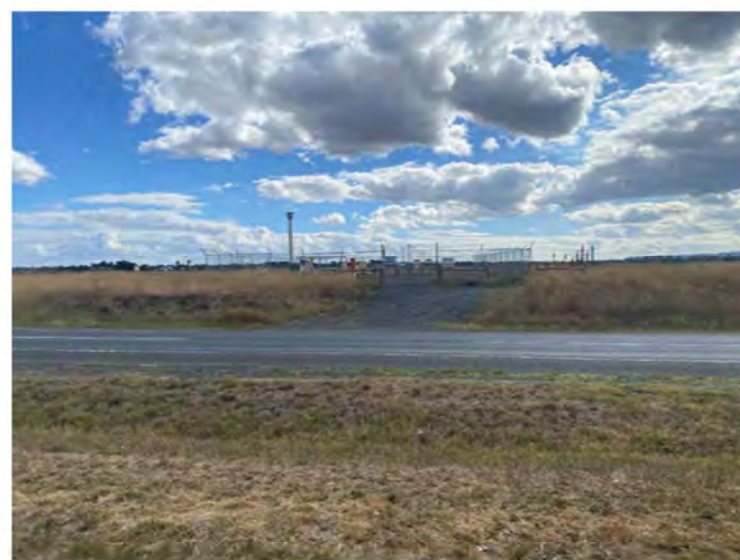
⑥ Infrastructure station abutting site
