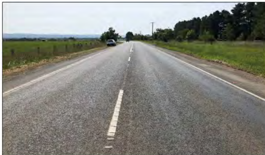
FIGURE 4: TRARALGON-MAFFRA ROAD FACING NORTH (SUBJECT SITE ON LEFT)
