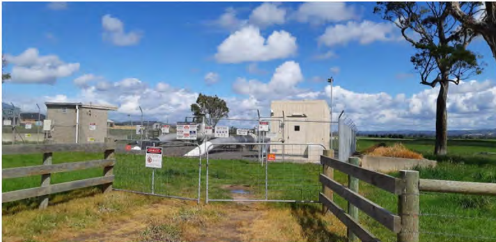
Plate 3: Gated entry to pipeline compound, looking west
