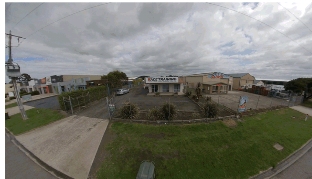
Rocla Road Street View
