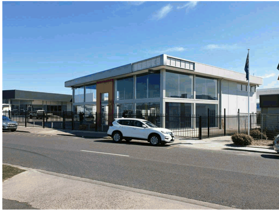
EXTERIOR VIEW - STREETVIEW LOOKING NORTH
