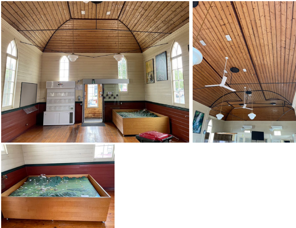
View of the interior looking toward the porch showing covered ceiling and steel rod collar tiles and non-original lights and fans. Note 'Diorama' in corner at right of left image, and bottom left
