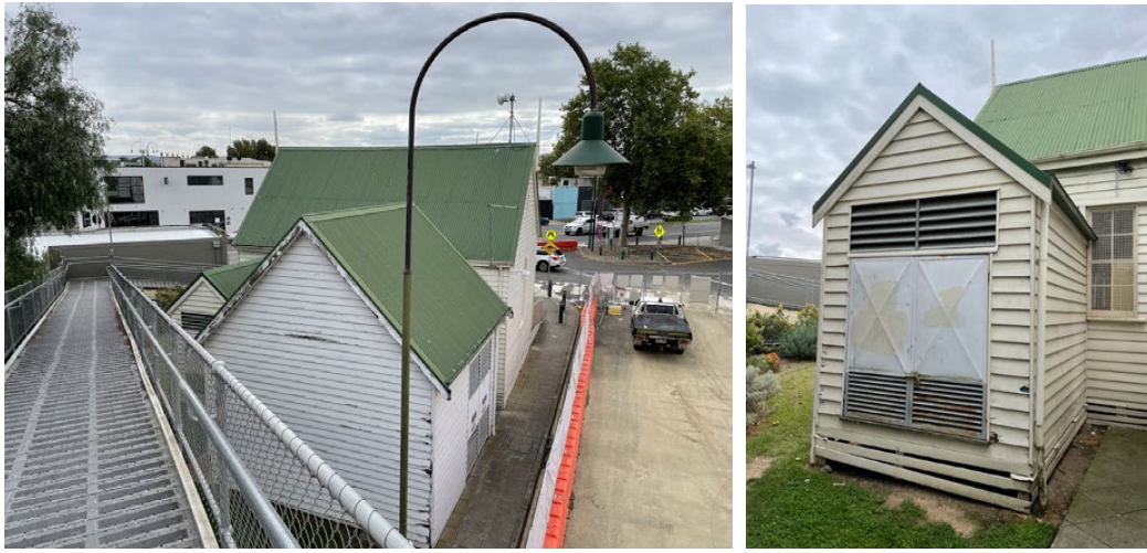
At left, view from pedestrian bridge showing substation at the rear. At right, non-original section added to the building upon relocation with non-original window at right.
