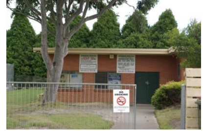
Tennis Courts Pavilion – no internal inspection as access was restricted.
