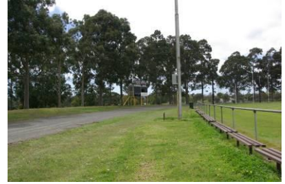
The boundary lines appear to 'cut in' and straighten along the wings. The boundary should be located at the road edge.
