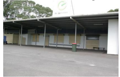
Football Pavilions – no internal inspection as access was restricted.
