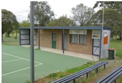
Netball Pavilion – no internal access. Pavilion externally appears in a reasonable condition.
