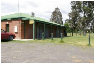
Cricket / Baseball Pavilion – no internal inspection as access was restricted. Shaded areas (veranda) appeared to be minimal and no clear access apparent from pavilion to oval.
