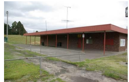
Drainage to be improved, including access around the main soccer pavilion.
