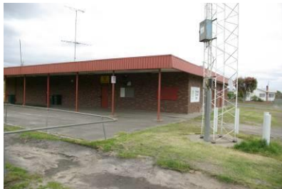
Monash Soccer Pavilion – no internal inspection as access was restricted.
