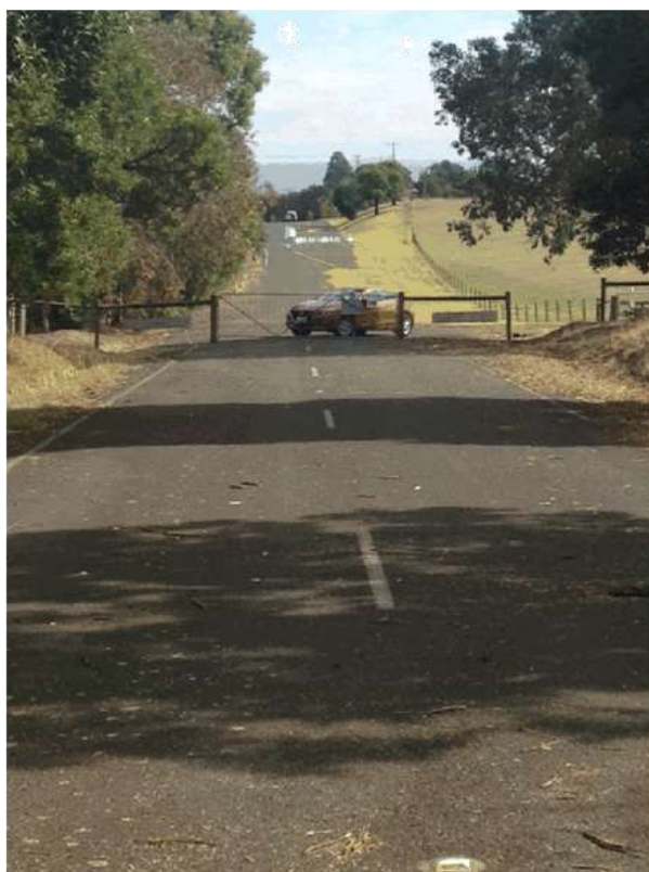
Photograph Two: Existing gate on Craighburn Place, Traralgon East, looking north.
