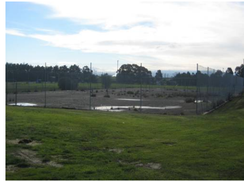
Figure 11: Inactive tennis courts
