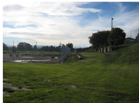
Figure 22: Embankment west of tennis courts
