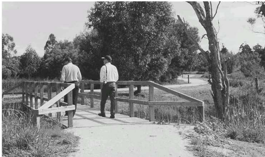
Walking path and bridge over Eel Hole Creek
