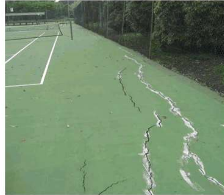
2. Looking west along northern boundary – long term cracking caused by adjacent trees.
