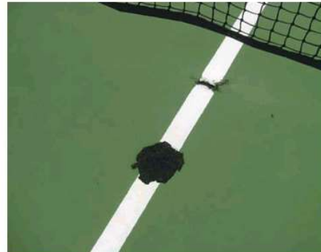
12. Typical patch over core sample taken from net on Court 15 – taken by Provincial Geotechnical on 6 th August 2012. Material was 25mm of Bitumen, over 110 crushed rock over 390mm of sand mix( bedding sand fill).
