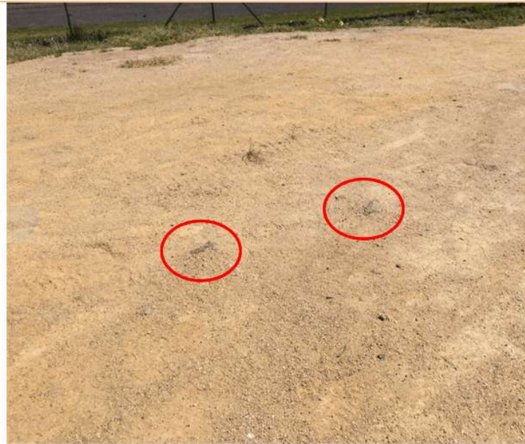
Image 4 – Pieces of recycled bitumen used as fill during track construction – Ronald Reserve, Morwell.
