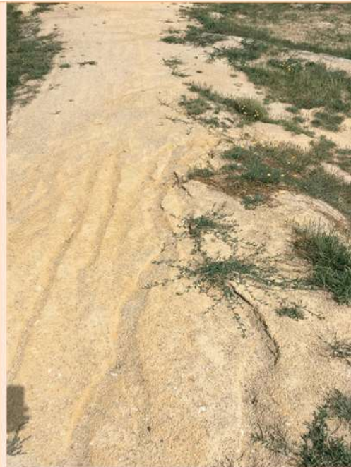
Image 3 – Close up of erosion on riding surface caused by draining water at Glendonald park, Churchill
