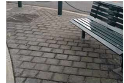
CONCRETE STENCILLING AND PRESSING
