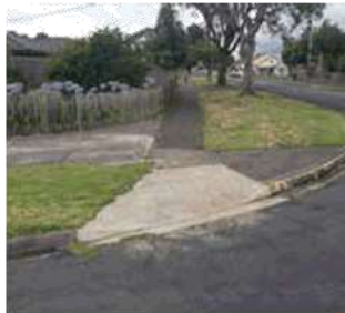
SINGLE RAMP- RECONSTRUCTED
