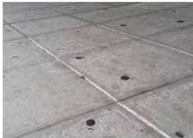
JOINTED CONCRETE PATH
