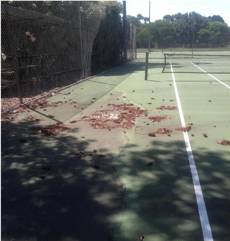
Careful consideration needs to be given to the existence of sports pavements immediately adjacent to trees and shrubs. Very rarely do they live in harmony together.
