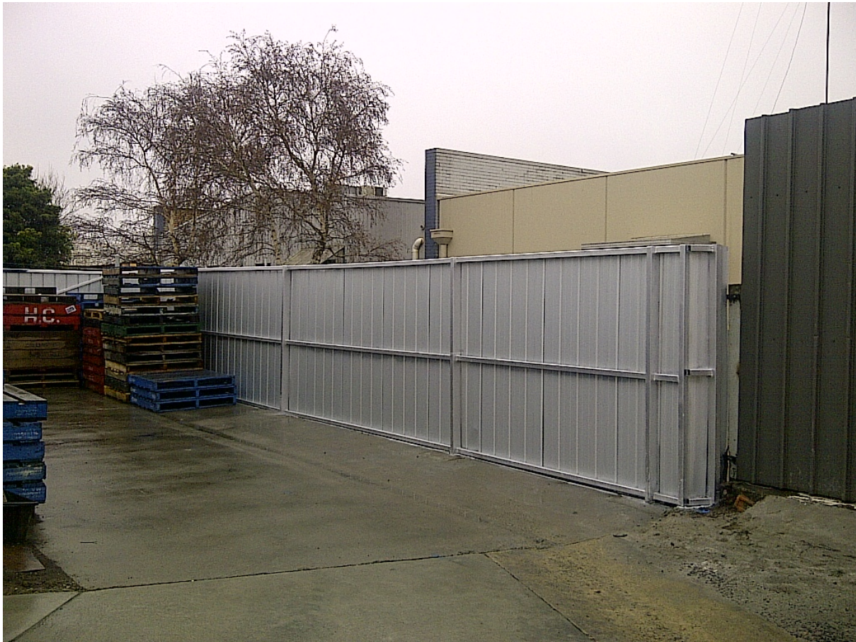
Permanent Fence Erected July 2013
