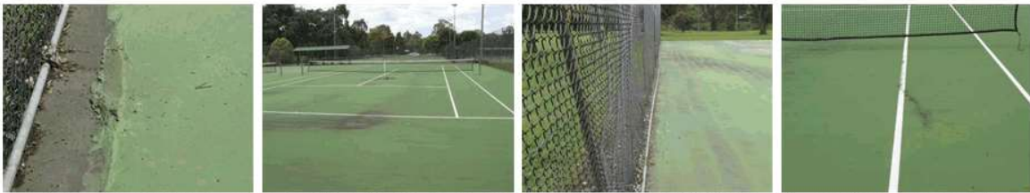
The worn and sub-standard acrylic surfacing can be replaced with a new and better quality material when applied.
