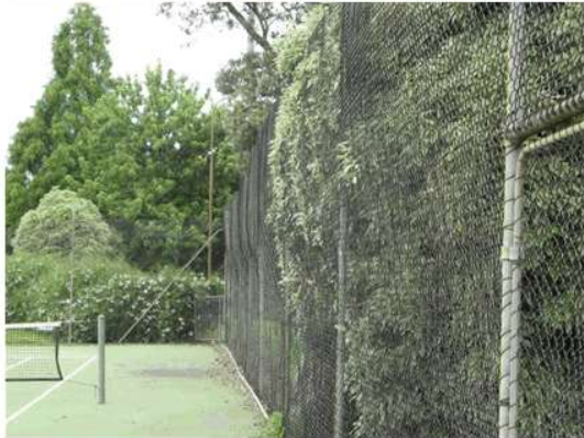
Large trees need trimming away from the court fencing to prevent damage to the fencing and to help minimise the amount of debris on the courts. Root barriers should be placed wherever trees are in close proximity to tennis courts to prevent the invasion of roots under the pavements.
