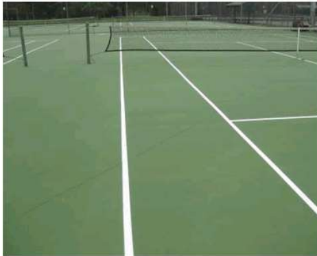
7. New tensile cracking to Court #3 following seismic event.
