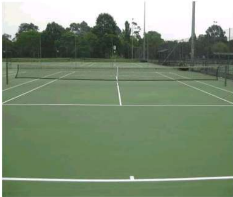
1. Typical view over tennis court # 3 – acrylic 'Laykold' top over original 'Rebound Ace' Synpave court.
