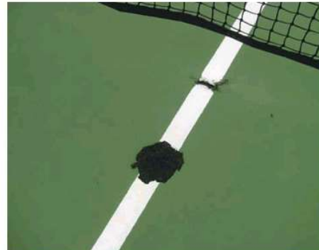
12. Typical patch over core sample taken from net on Court 15 – taken by Provincial Geotechnical on 6 th August 2012. Material was 25mm of Bitumen, over 110 crushed rock over 390mm of sand mix( bedding sand fill).
