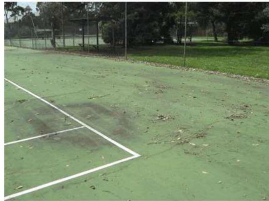
Damage to the courts due to tree root invasion and poor drainage is consistent across all courts in the facility.
