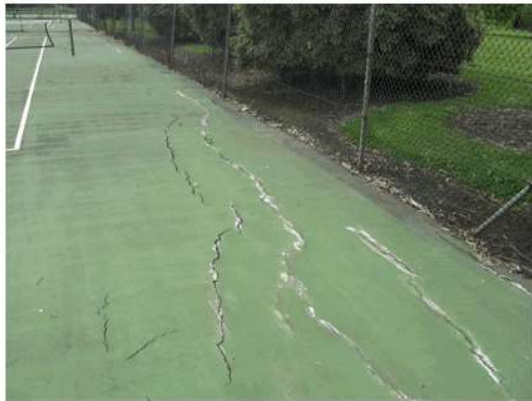
Damage to the courts due to tree root invasion and poor drainage is consistent across all courts in the facility.
