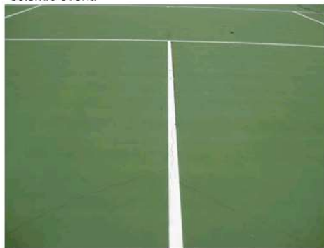
9. Long term crack on court # 6, existing crack has propagated further following the seismic event.
