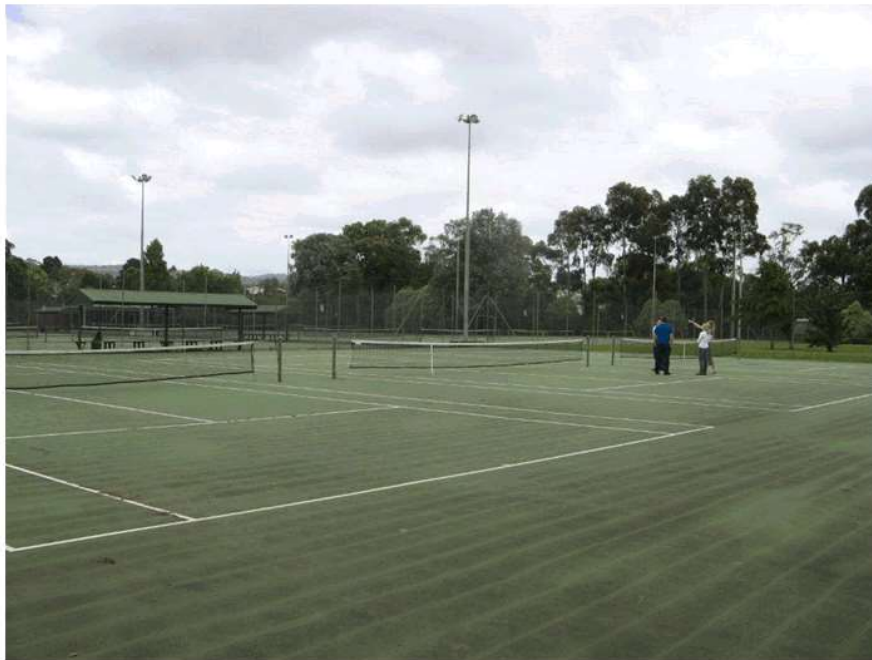
Figure 2 – Typical Court Condition
