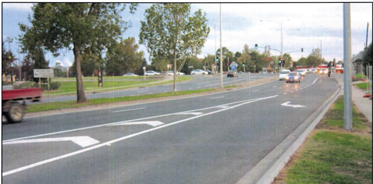
Figure 3-3 Princes Highway facing South
