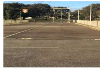
Fire Brigade training track
