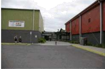
Main entry to stadium. No designated drop off zone or accessible parking within 20.0m of entry.
