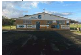
View of sports pavilion from the car park. Car parking recently sealed. Need to delineated car parking spaces
