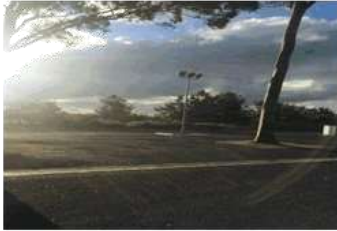
Henry Street Car Park with lighting and drainage
