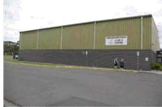
Existing stadium (southern courts) appears in a reasonable condition. Evidence of wear and tear at close inspection.
