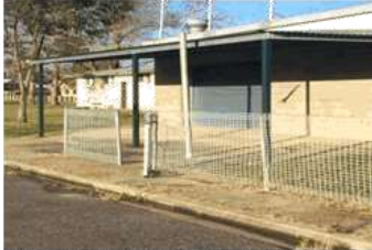
Fire Brigade storage shed and kiosk
