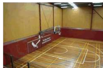
Safety run-off for both netball and basketball not to sports specifications.
