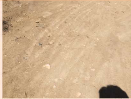
Image 6 – Recycled Bitumen and Stones used in track construction – Ronald Reserve Morwell
