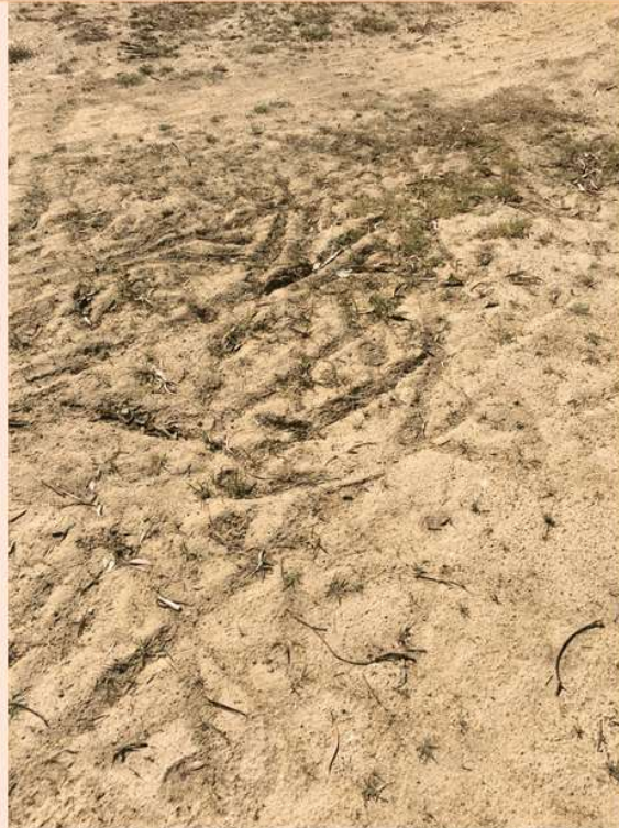
Image 7 – Erosion/Water Pooling damage caused to riding surface - Newborough
