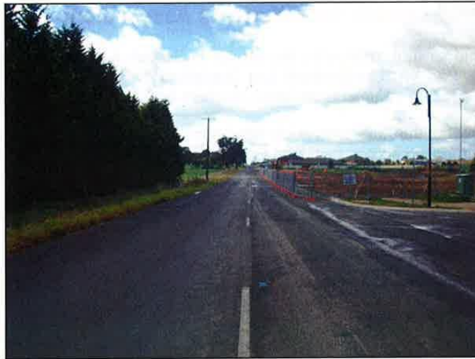
Photo 7: Cross's Road at proposed Access Point 1, looking east
