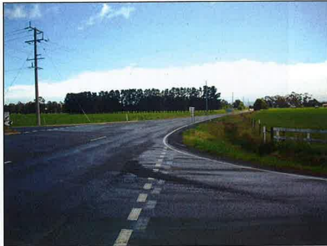
Photo 4: Tyers Road, looking north from Cross's Road
