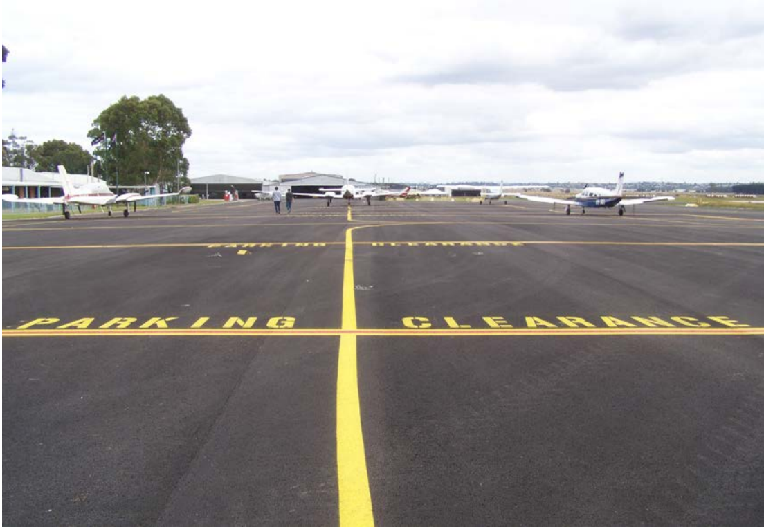
(Pictured above – Main Apron Area Refurbishment)
