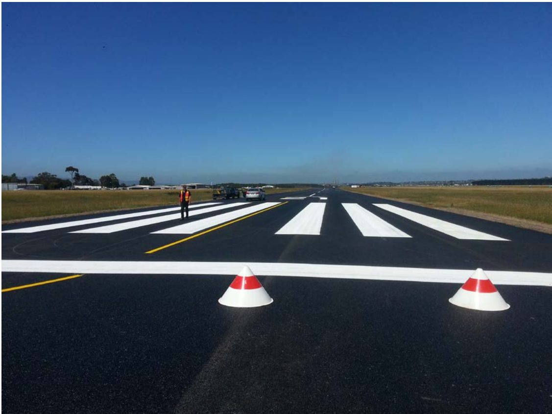
(Pictured above: Sealing of the main runway 03/21)
