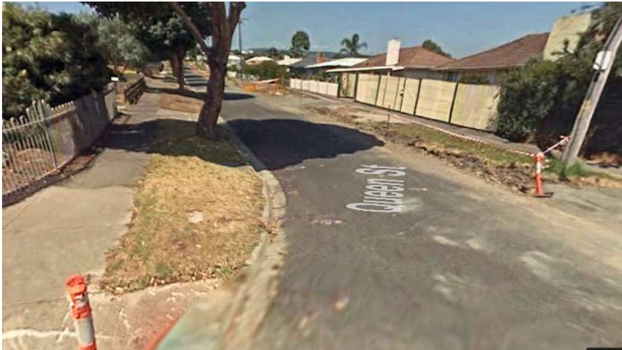
Figure 1 – 39 Queen Street verge during construction
