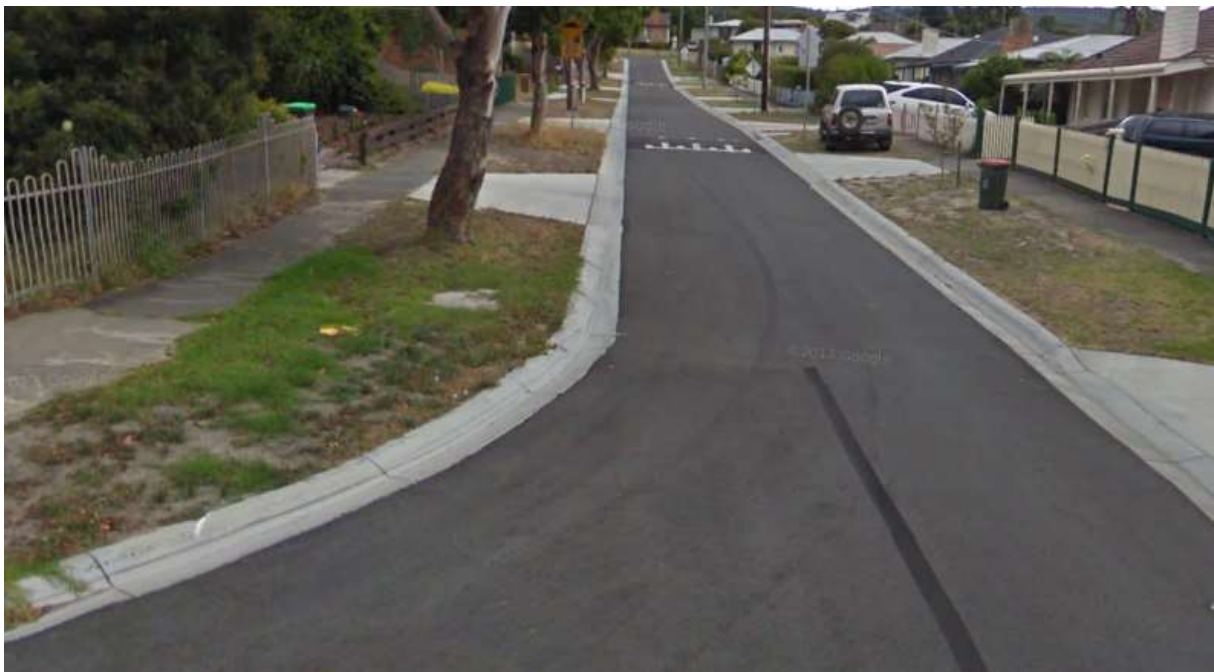
Figure 2 – 39 Queen Street verge after construction
