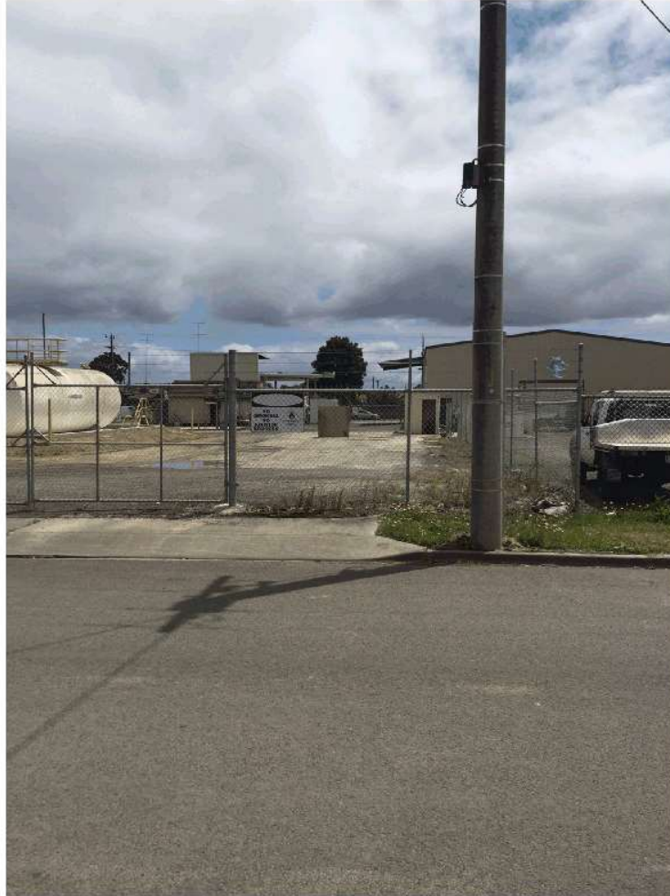
Photograph 2: Middle section of discontinued laneway incorporated into 23-29 Shakespeare Street, Traralgon.
