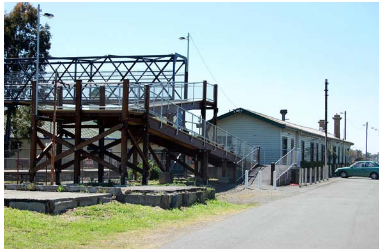
Repurposed station building and pedestrian overpass
