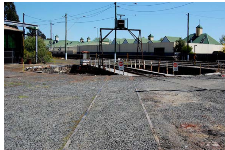
Heritage listed railway turntable
