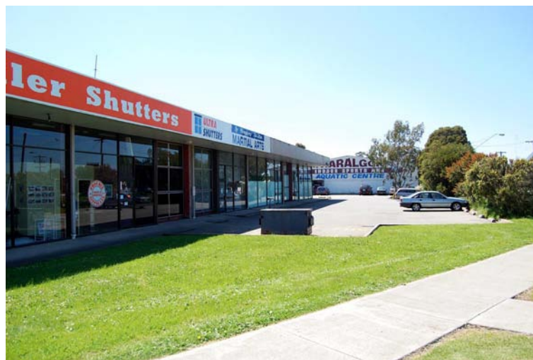
Existing commercial premises to west
