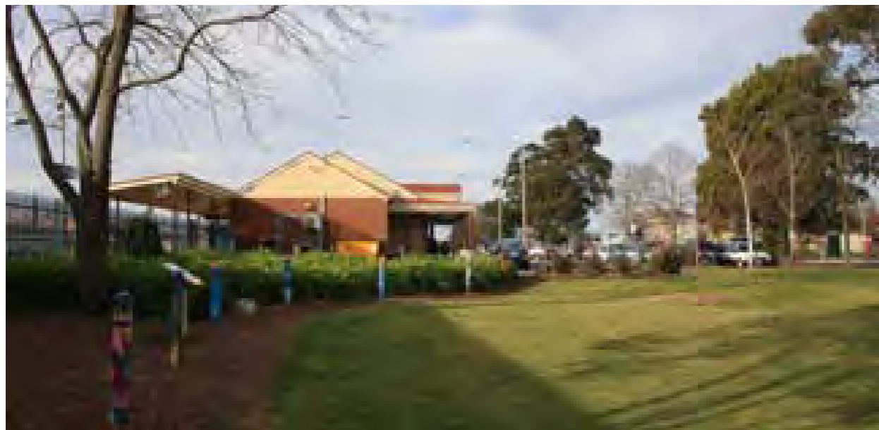
Existing Moe Train Station building and platform
