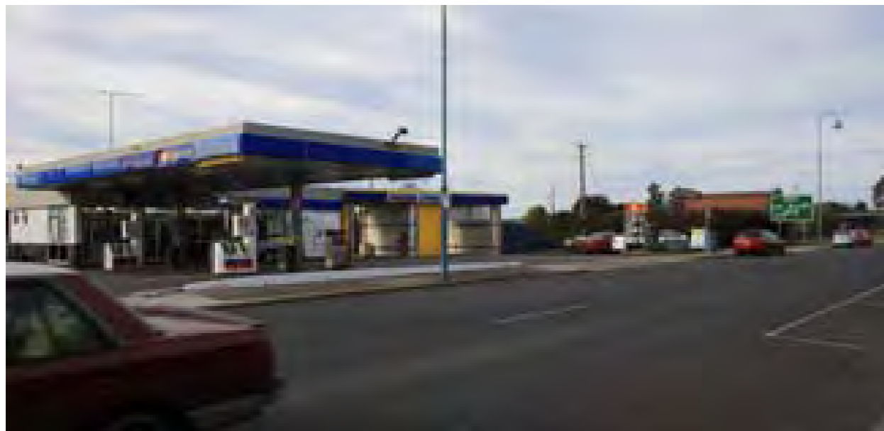
Existing Service Station within the Rail Precinct, on Lloyd Street
