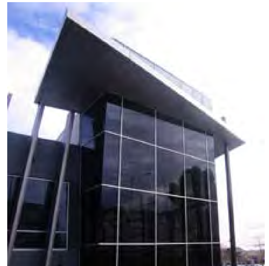
The Hume Global Learning Centre in Broadmeadows contains a library, gallery space, cafe and computer facilities, providing a vital civic hub function.
