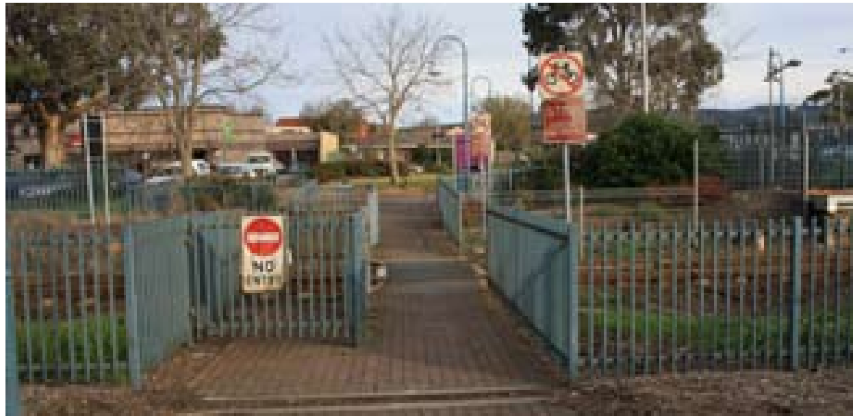
Existing pedestrian level crossing, looking south towards Lloyd Street
