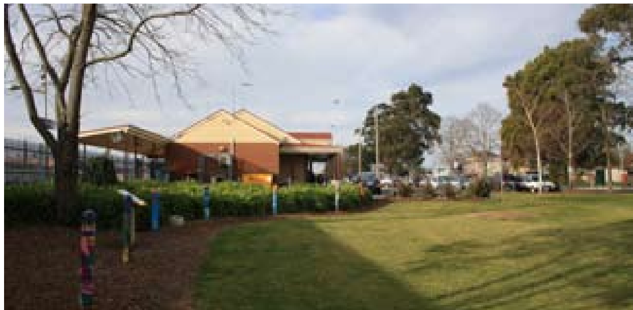
Existing Moe Train Station building and platform
