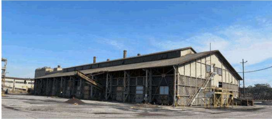
View southwest to Briquette Storage Shed.
