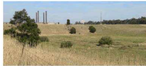
Ancillary land surrounding Morwell Power Station and Briquette Factories
