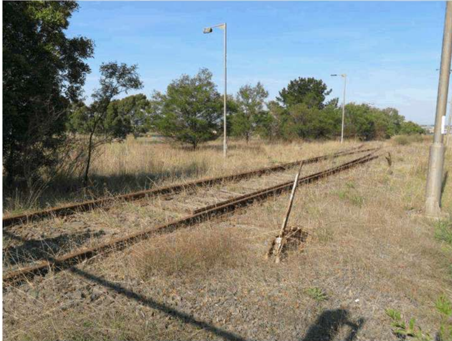
Rail siding connecting to Briquette Loading Station, looking southeast.
