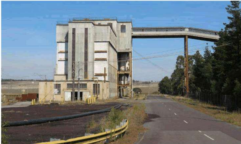
Raw Coal Bunker
