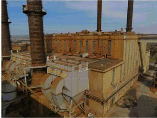
Power Station Boiler House
