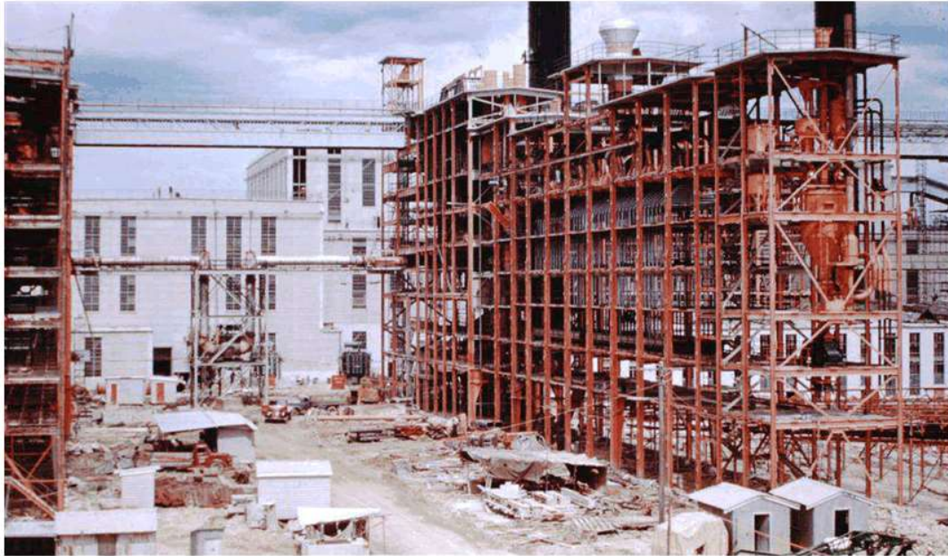
Construction of the Briquette Factories, undated. (Source: http://ebacdemolition.com.au/about-history/ )
