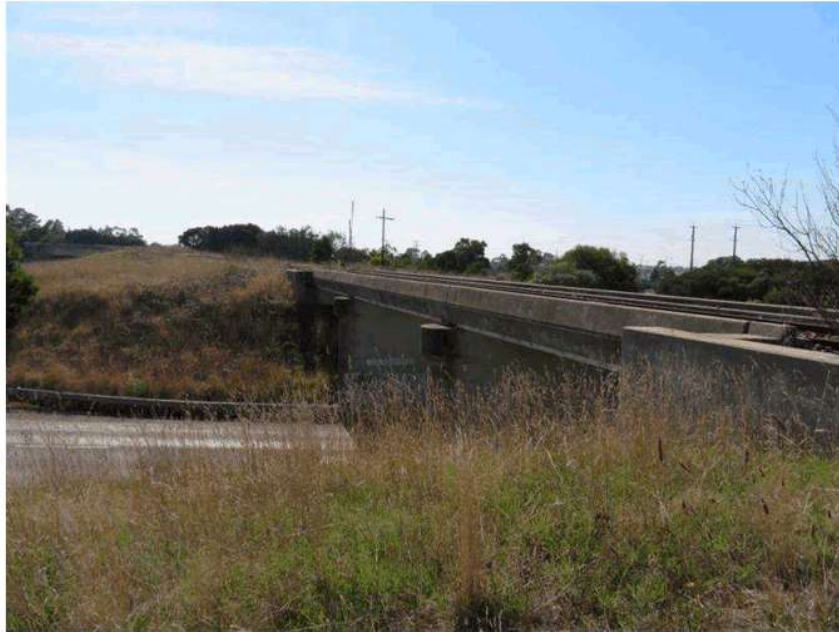
Commercial Road railway overbridge, looking northwest.
