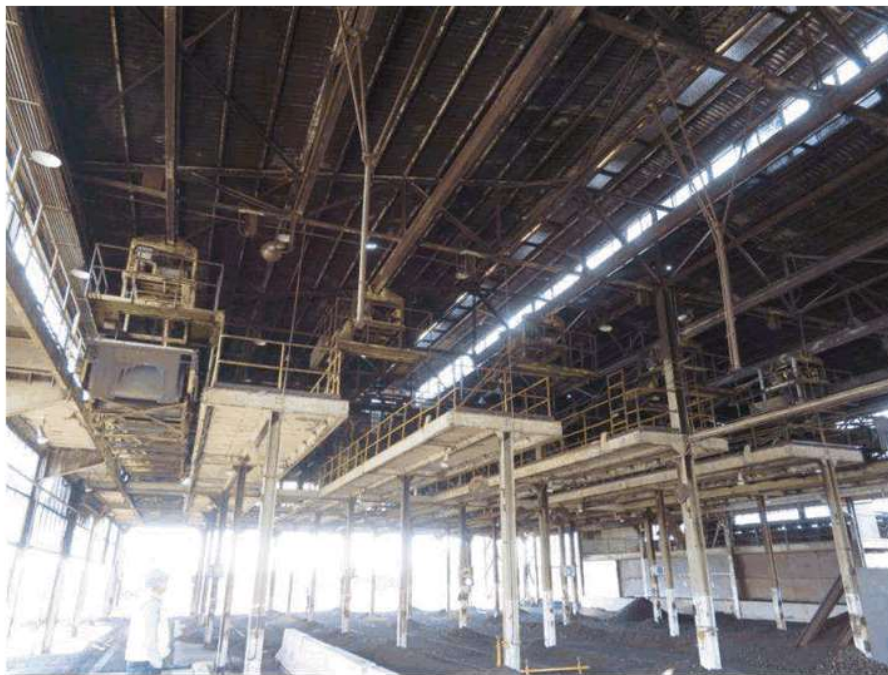
View from under the briquette loading station.
