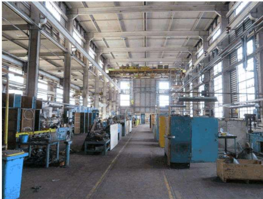
View inside the Mechanical Workshops, looking east.
