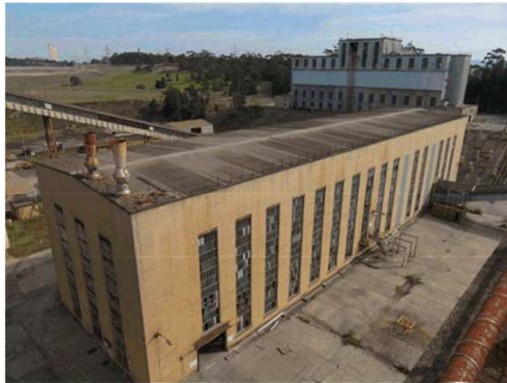
Wet Section Building
