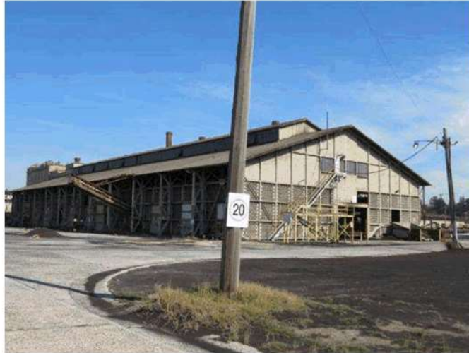
Briquette Storage Shed
