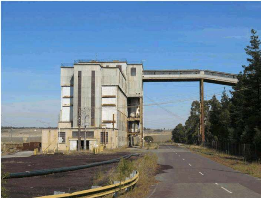
View south to the raw coal bunker and conveyor.
