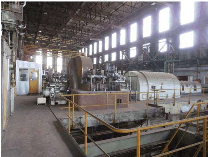
View inside the Turbine House, looking northeast.
