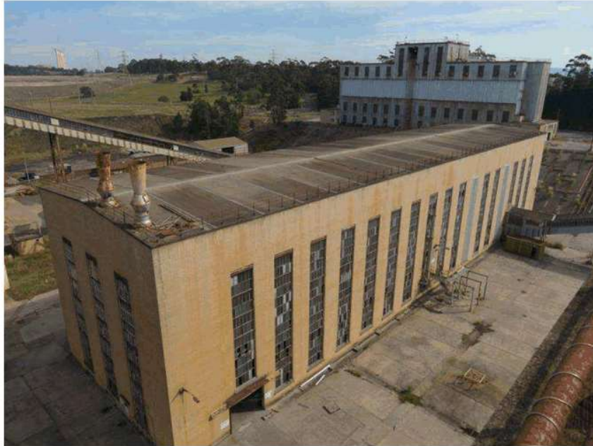
View southwest from the top of No.1 Briquette Factory looking at Wet Section No.1 building (foreground) with the raw coal bunker visible (background)
