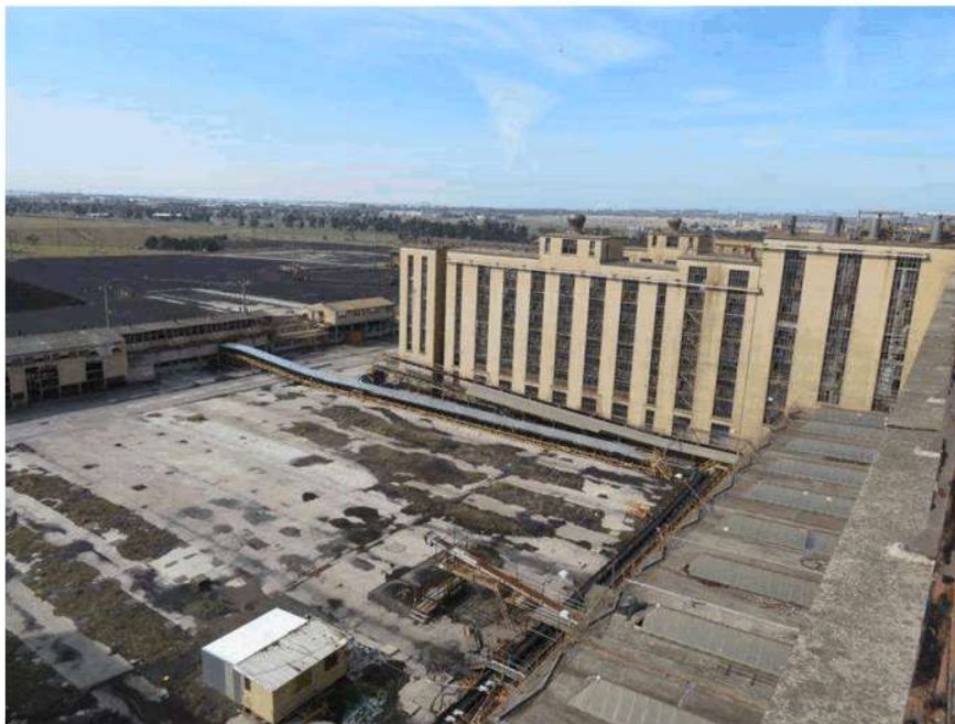
View northeast from the top of No.1 Briquette Factory looking at side of the Briquette Factory (right) and the collecting and feeding conveyors (left)
