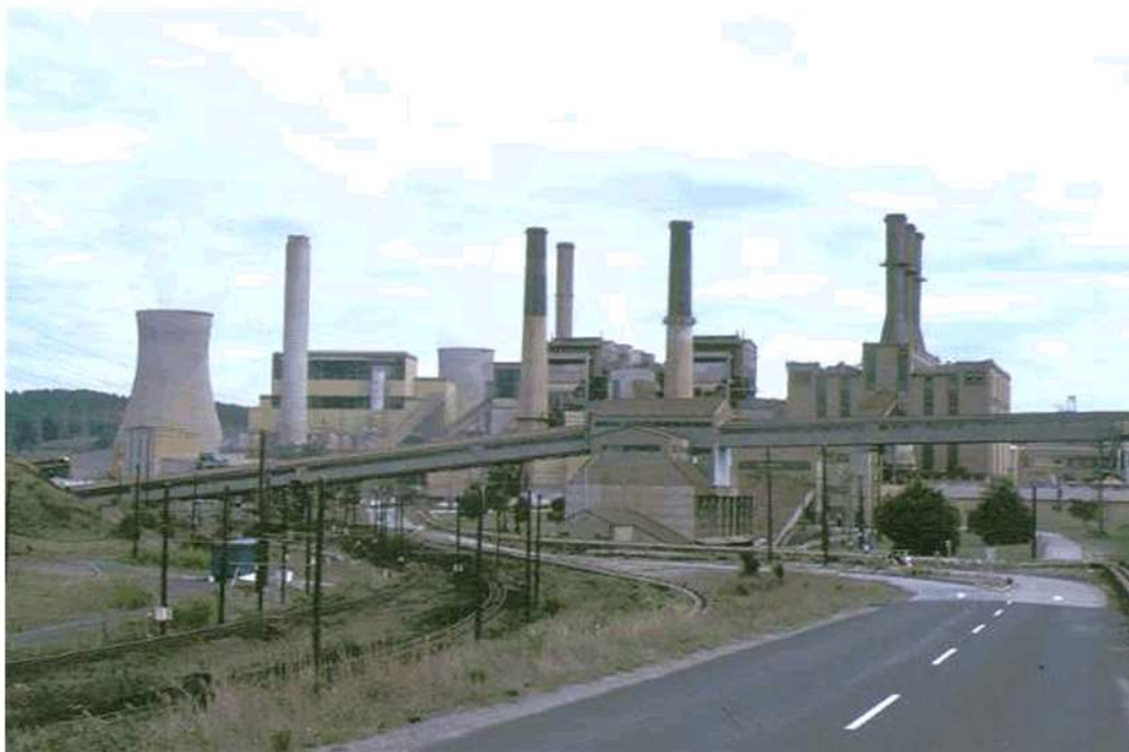
Yallourn Power Station (VHR H1054) (demolished)
