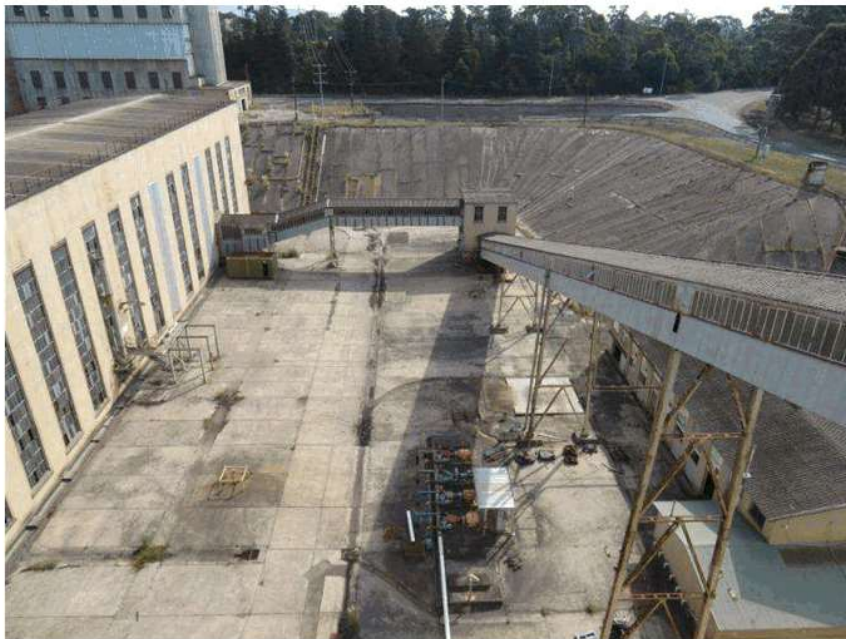
View east from the top of No.1 Briquette Factory looking at the conveyors and North West Corner Station.
