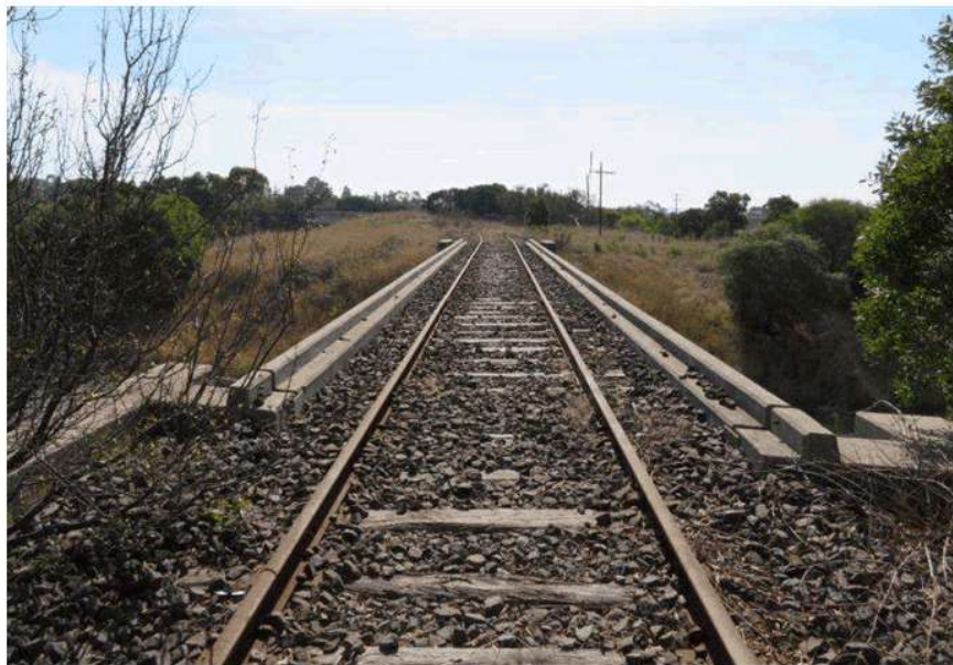
View north along Commercial Road overbridge to the north.
