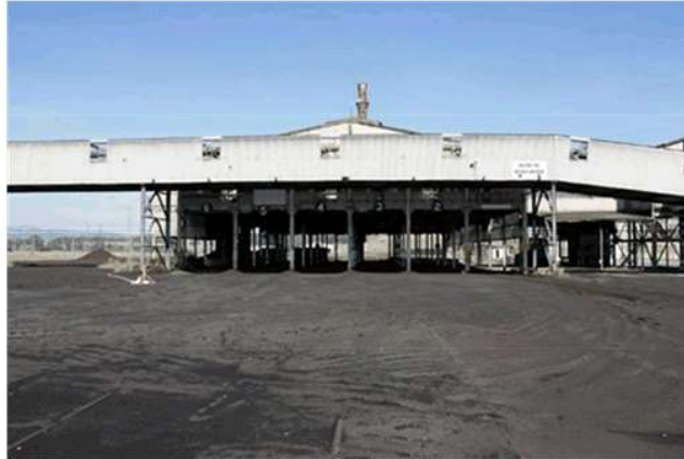
Briquette Loading Station
