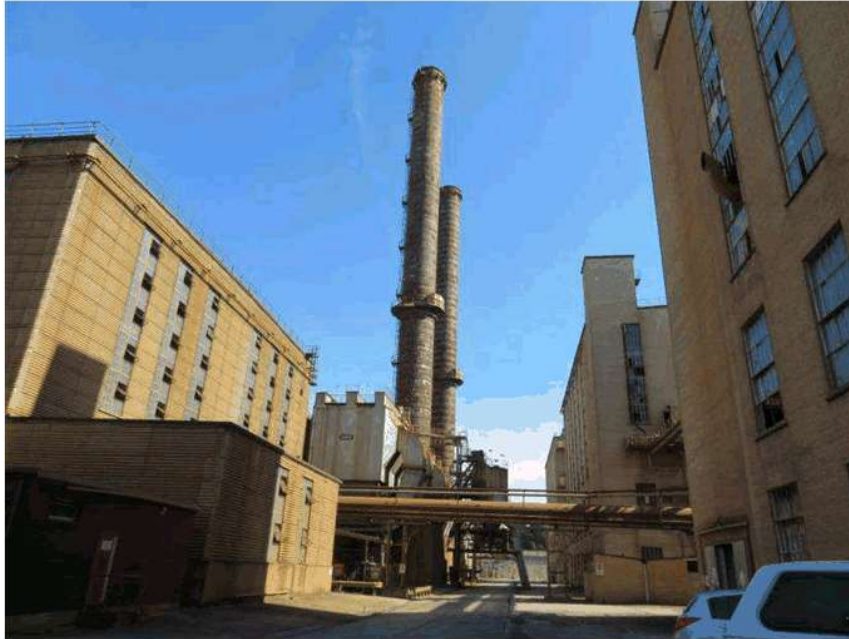
View looking west between Briquette Factories (right) and Power Station with chimneys 3 and 4 (left).
