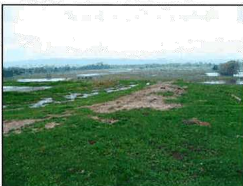
Plate 9: View NE from top of slope where 240 Cross's Road AS (8221-0182 [VAHR]) is located.
