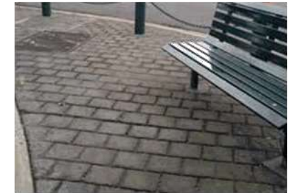
CONCRETE STENCILLING AND PRESSING
