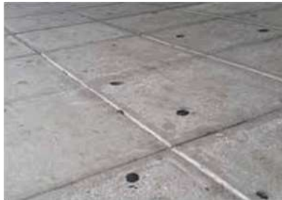
JOINTED CONCRETE PATH
