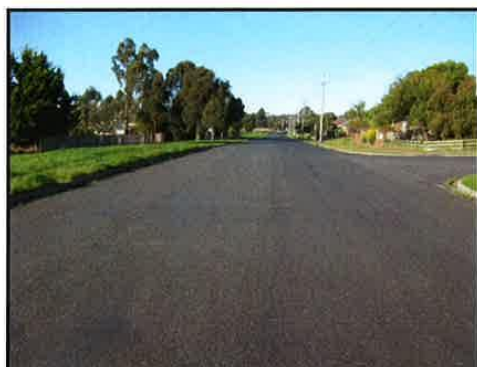
Photograph 1: Acacia Way - View East
