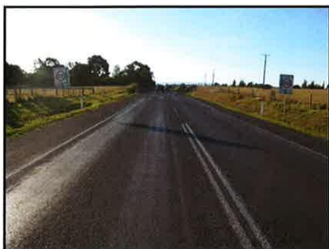
Photograph 3: Monash Way - View North
