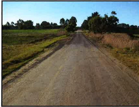
Photograph 5: Silcocks Road (North-South Leg) - View North
