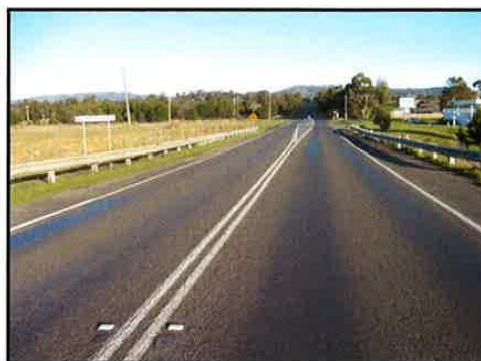
Photograph 4: Monash Way - View South
