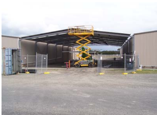
New production hangar
