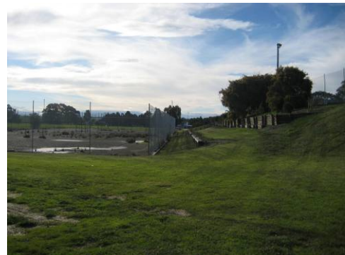
Figure 22: Embankment west of tennis courts
