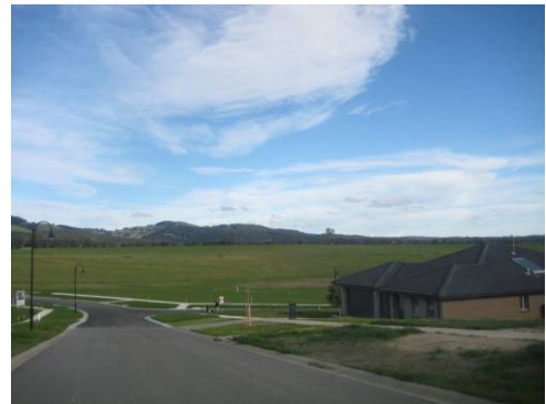
Figure 2: Residential development frontage
