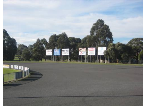
Figure 20: Sealed asphalt road around main oval
