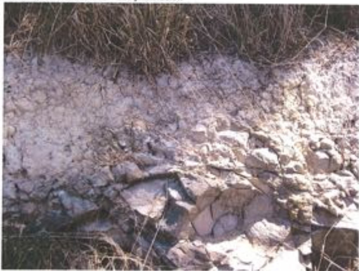
Photo 2: Soil in subject area – weak clay/silts over soft rock.
