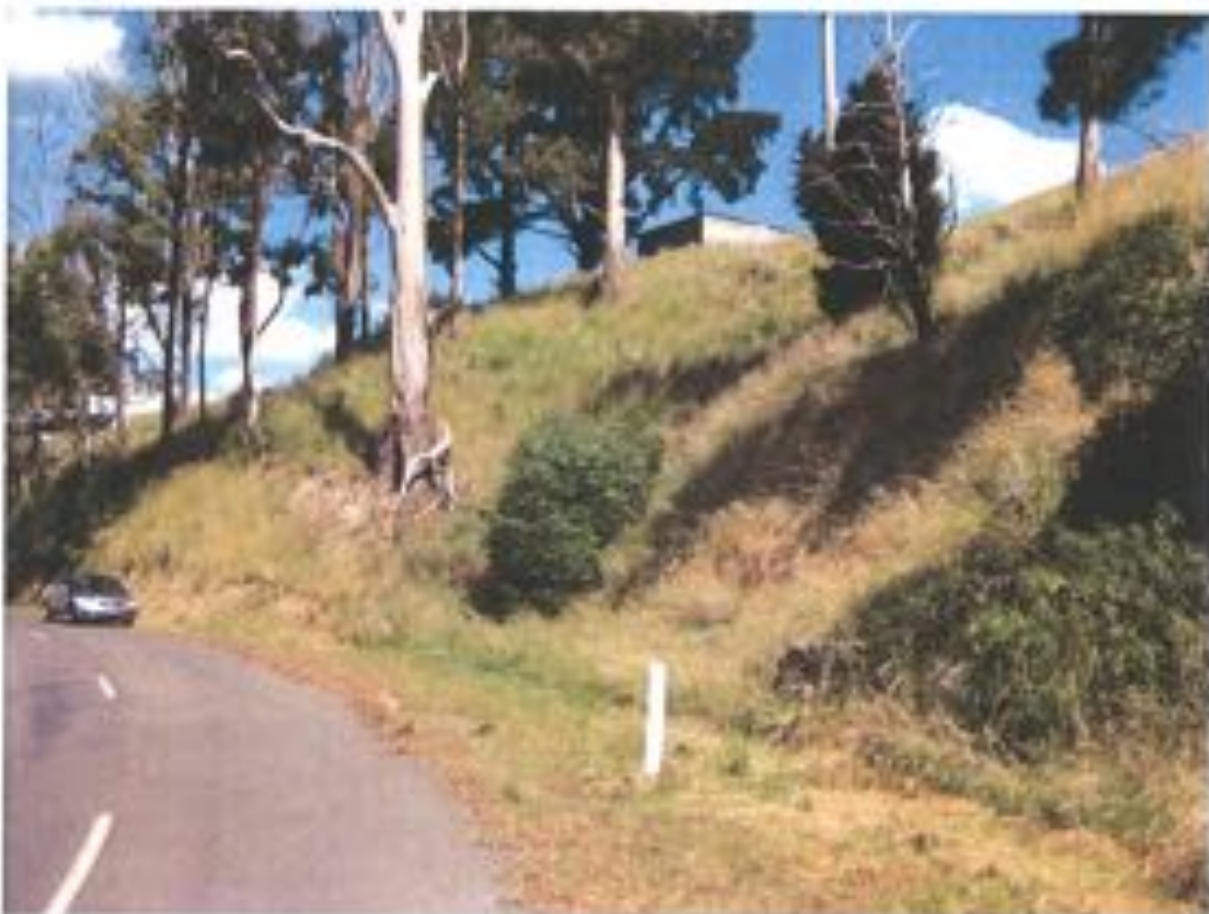
Photo 3: Site of most recent landslide approx 4 years ago – this event blocked the road, cutting access- this is approx 200m west of the proposed works ie similar soil and
