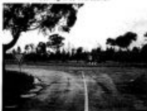
Figure 4 - Northern Avenue looking southeast to the Princes Highway intersection
