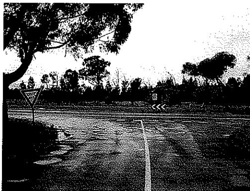
Figure 4: Northern Avenue looking southeast to the Princes Highway intersection
