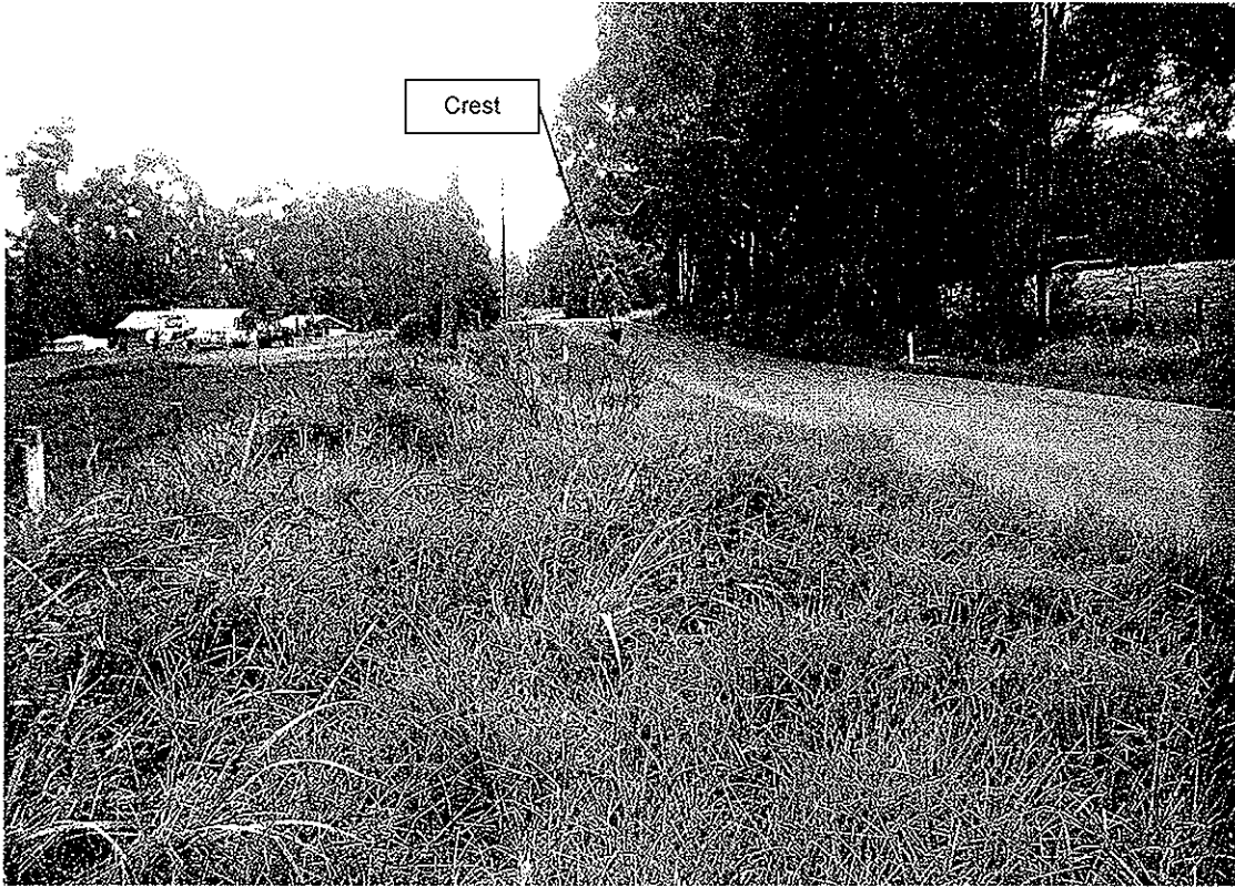
View of the subject site, looking to the north (The sight distance at the northern end of Lot 2 is impeded by a crest in Two Mile Road as shown above)
