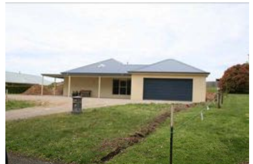
New residential development around the precinct.
