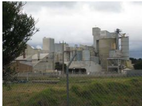
Unimin Traralgon Plant.
