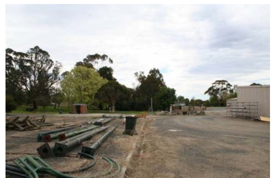
The existing Traralgon Depot site.
