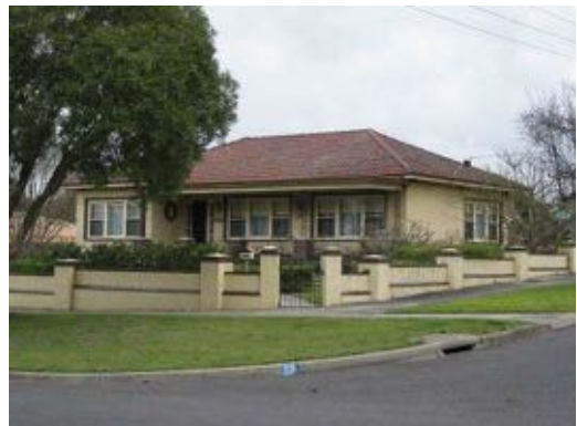
Existing single storey residential adjacent to the precinct.
