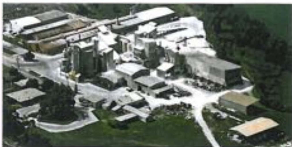
Existing Plant Looking from the South West
