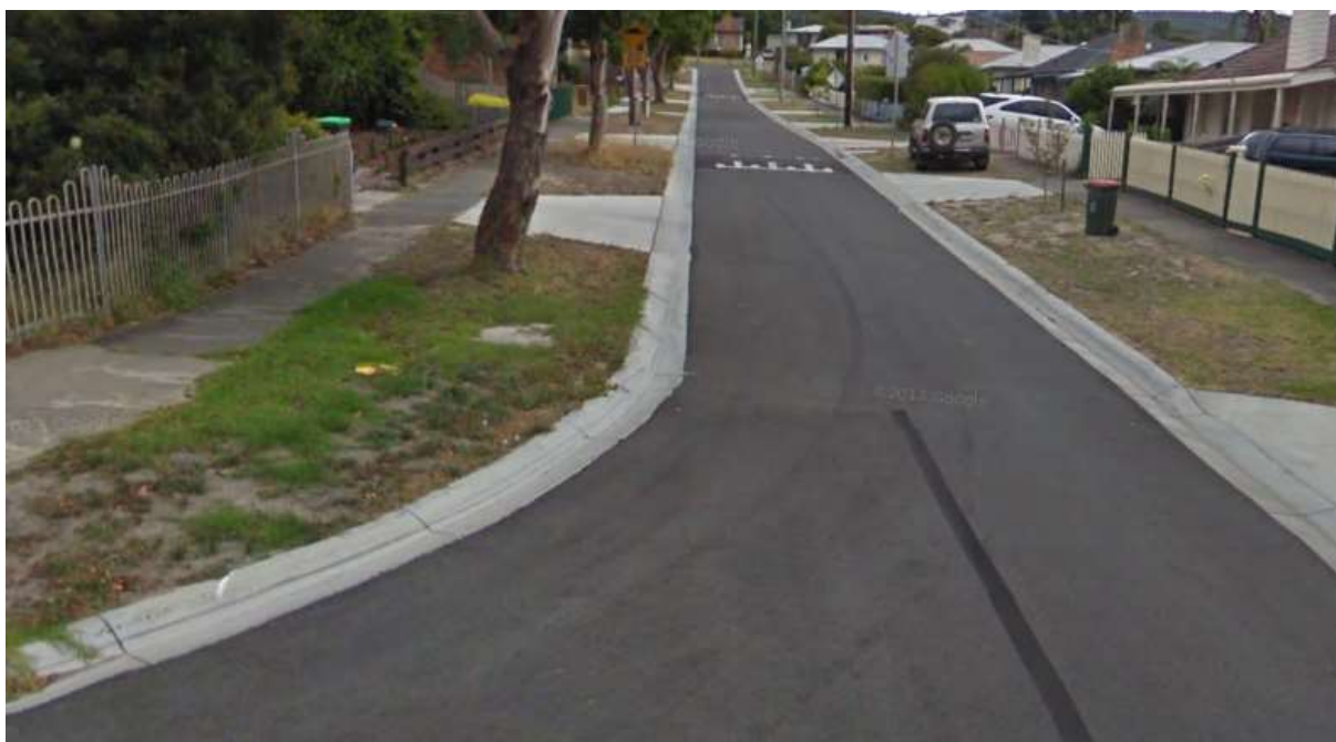
Figure 2 – 39 Queen Street verge after construction
