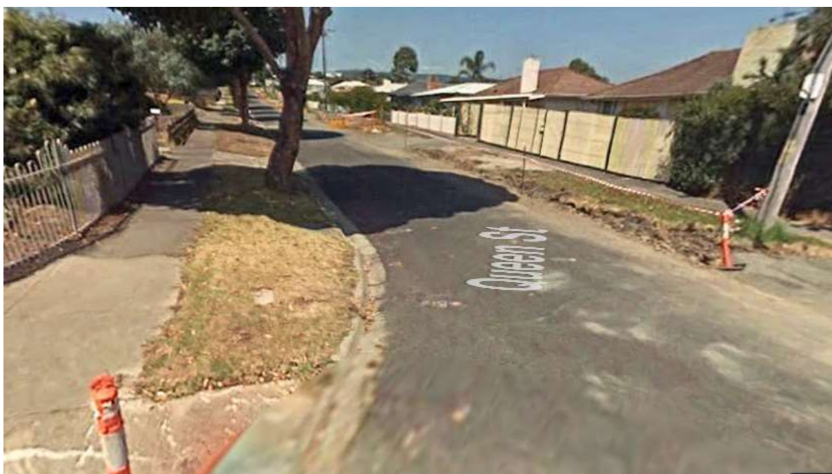
Figure 1 – 39 Queen Street verge during construction
