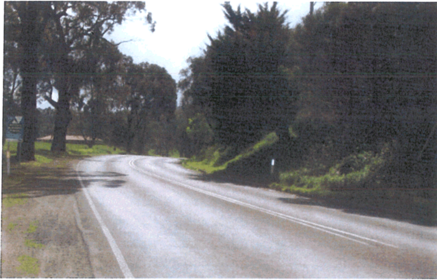
Photo 3: Walhalla-Tyers Road, looking north to sharp bend
