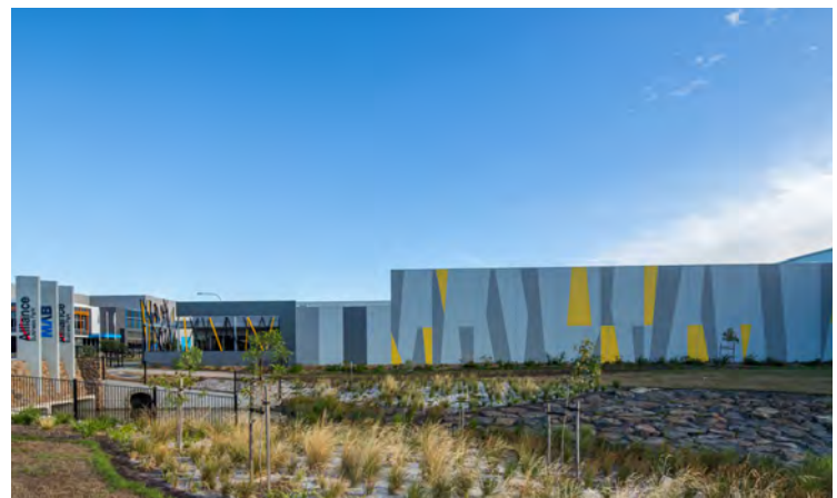
Example of a well-oriented industrial building with integrated WSUD initiatives
