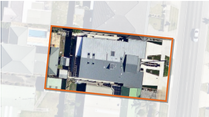
Example of typical townhouse development in Traralgon
