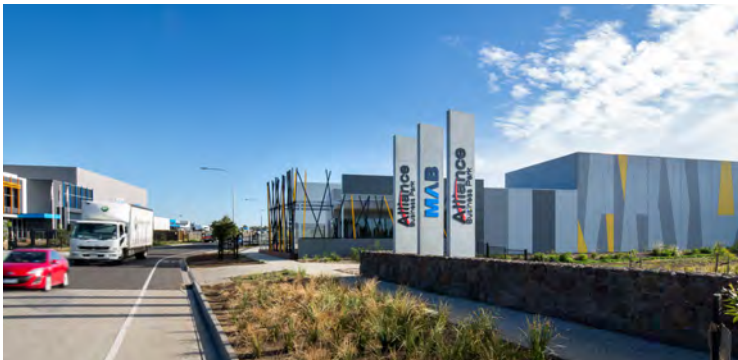
Example of sealed pedestrian path
