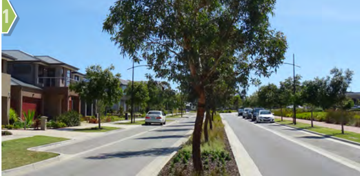
1 Example of inset car park car parks and central median to slow traffic speeds
