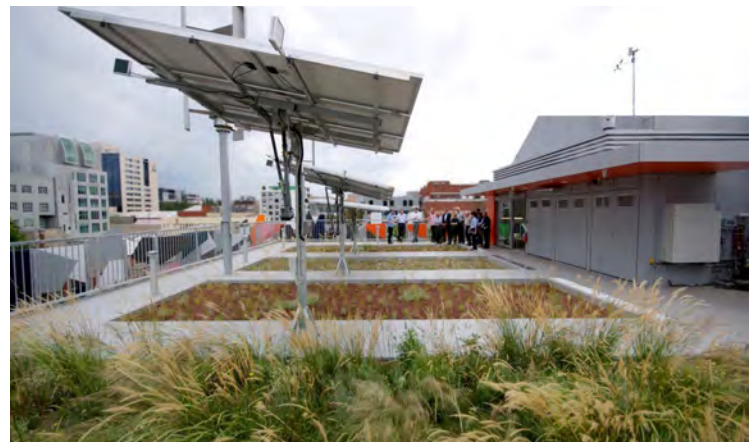
Example of commercial rooftop incorporating solar panels and landscape
