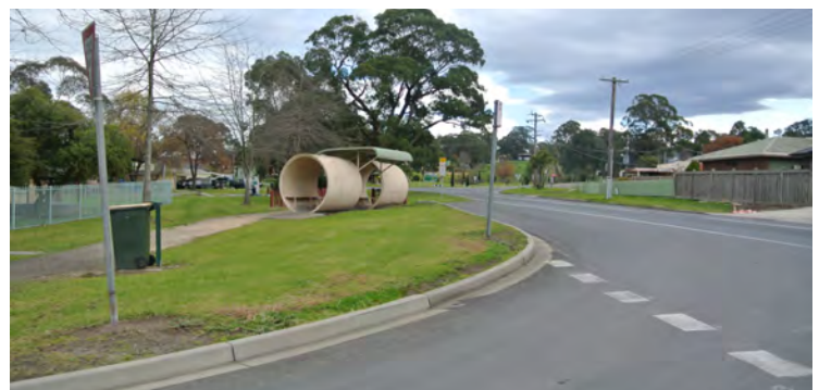
Existing street condition common in Tyres
