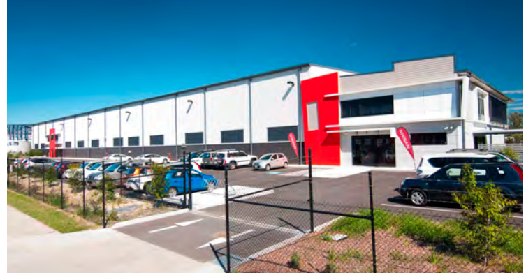
Example of a security fence to the street
