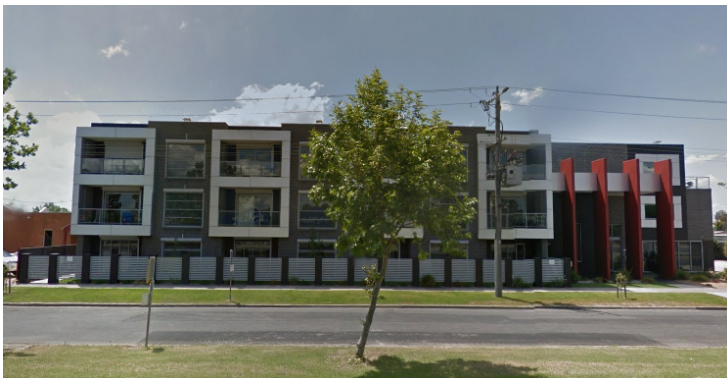
View of existing apartment typology in Traralgon
