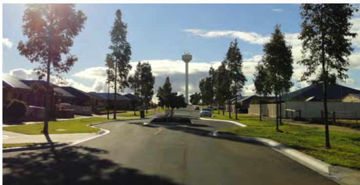
Example of collector street comprising traffic calming measures and wide nature strips
