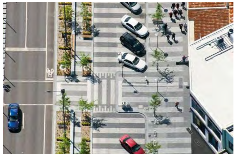
Example of pedestrian crossing (and integrated shared zone) in a commercial setting
