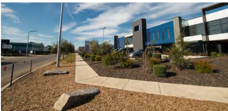
Example of sealed pedestrian path
