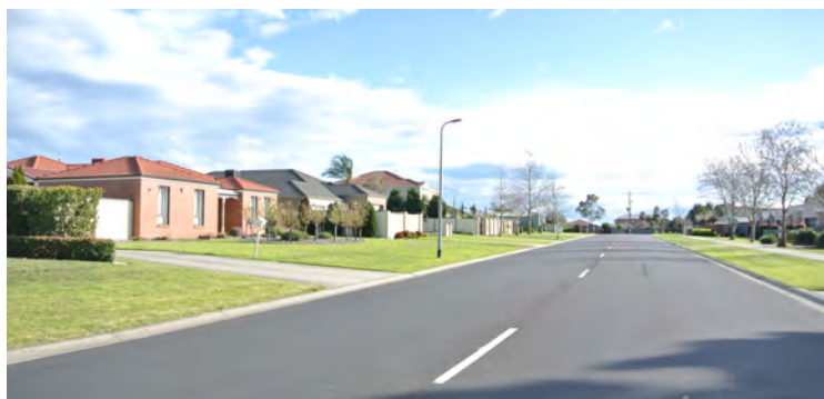
Existing residential street condition common in Traralgon
