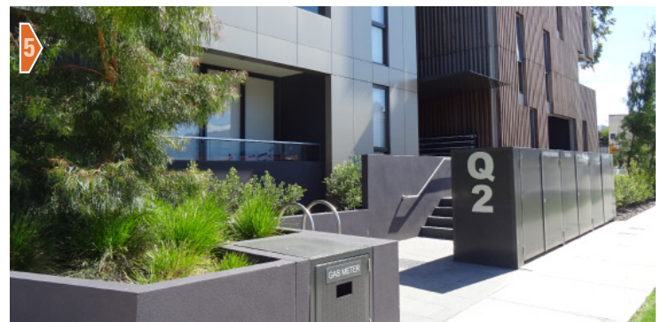
Example of booster cabinet integrated into street fence
