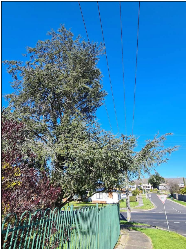
Figure 10: T5, lopping around powerlines.
