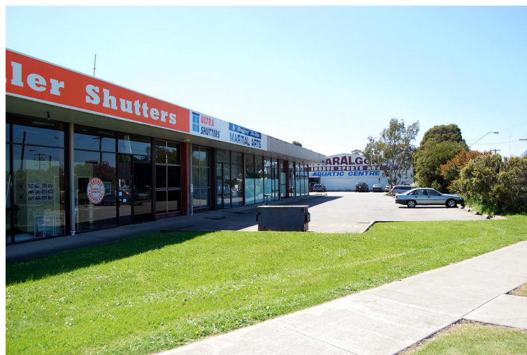
Existing commercial premises to west
