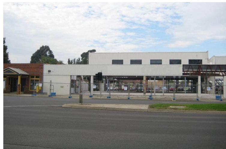
GippsTAFE building under construction
