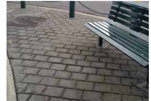
CONCRETE STENCILLING AND PRESSING
