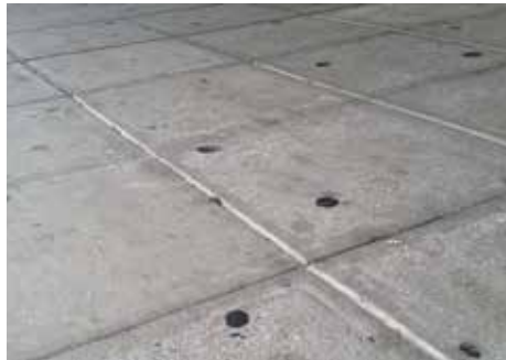
JOINTED CONCRETE PATH
