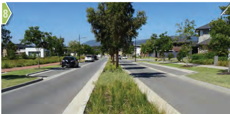
Example of paved and concrete footpaths within residential street context
