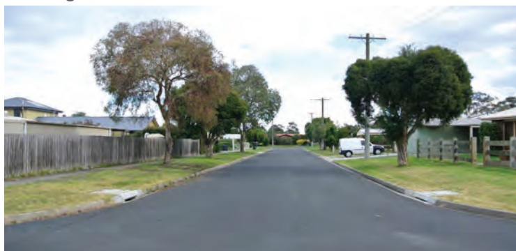
Existing residential street condition common in Glengarry
