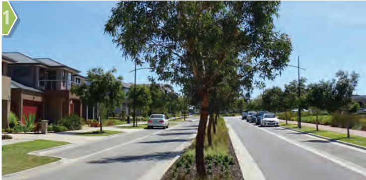
Example of inset car park car parks and central median to slow traffic speeds
