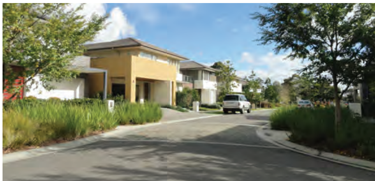
Cobble paving at street entries to slow traffic movement
