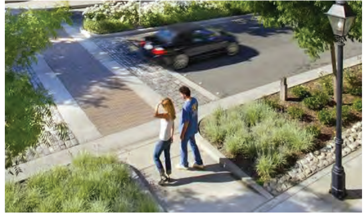
Example of pedestrian crossing defined by landscape and pavement
