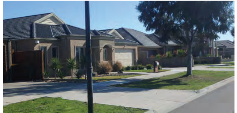
Typical footpath construction comprising a sealed, even surface.
