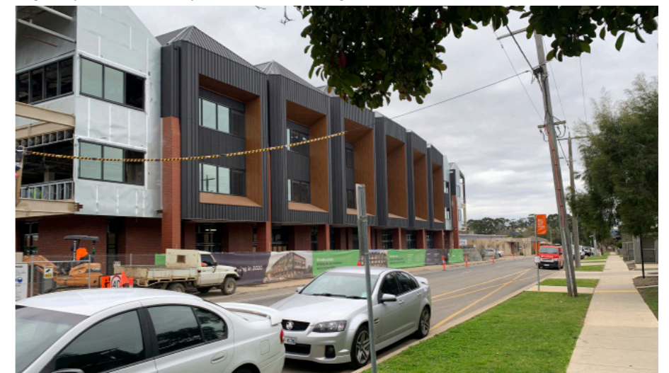
The GovHub building nearing completion
