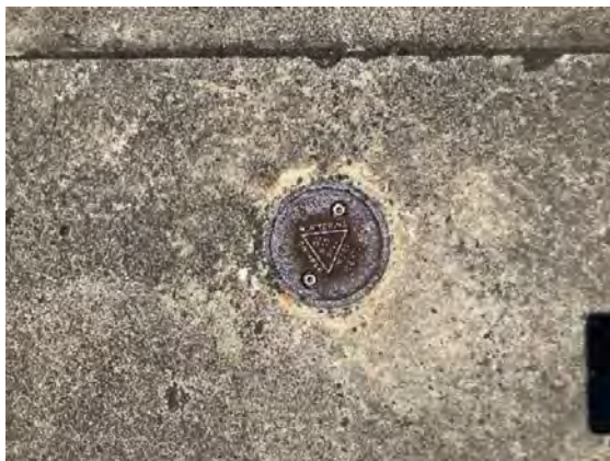
Image: LCC 30 Nov 2021 Water Well
