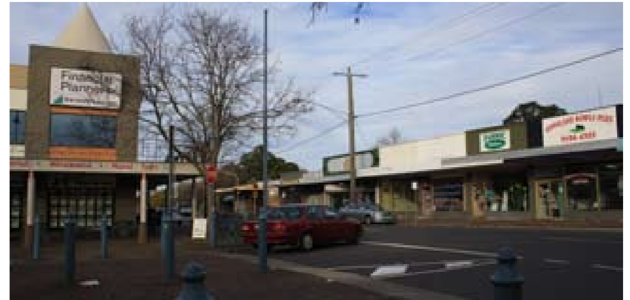
Intersection of Moore and George Streets, with Rail Precinct behind shops at right
