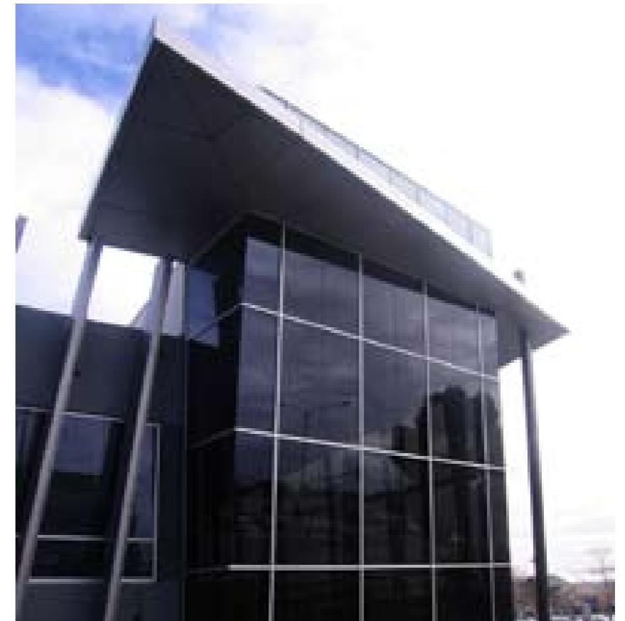
The Hume Global Learning Centre in Broadmeadows contains a library, gallery space, cafe and computer facilities, providing a vital civic hub function.
