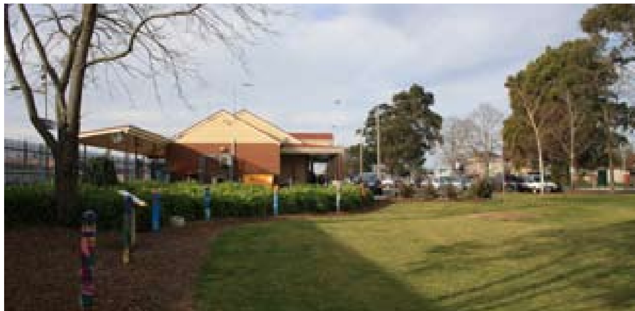
Existing Moe Train Station building and platform
