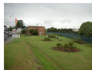
6. Potential for adaptive re-use of substation building adjacent rose garden and reserve
