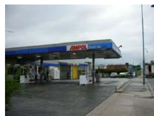
2. Existing service station site for redevelopment
