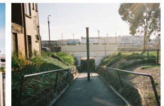
Existing pedestrian underpass
