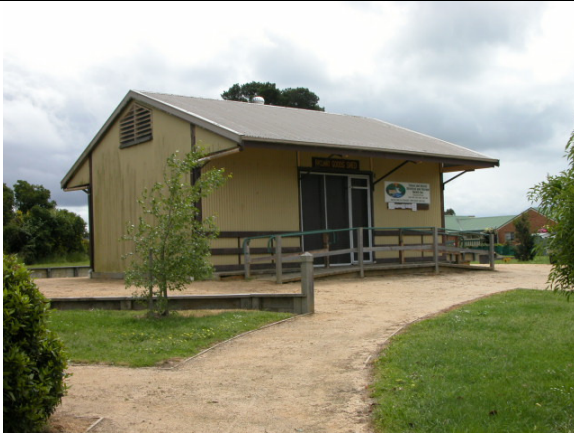
Yinnar Railway Station Goods Shed Source: Context, 2005
