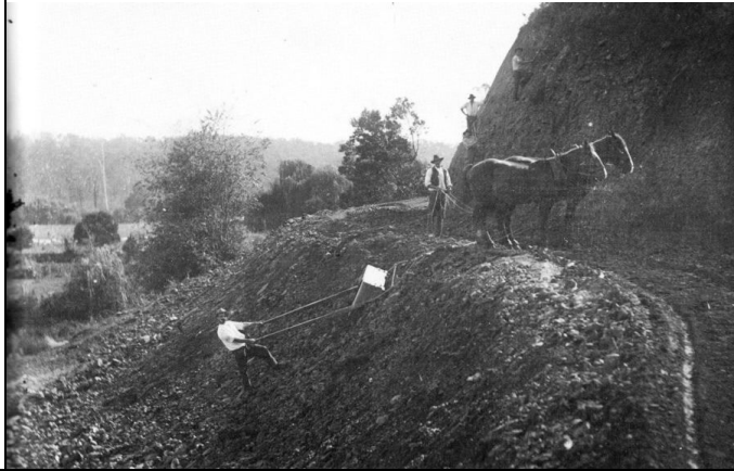
Using a horse scoop to construct Middle Creek Road, c.1900s
