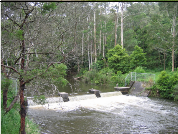
Traralgon Water Trust Weir, Latrobe River Source: Context, 2005
