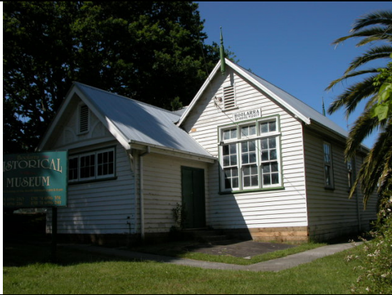
Boolarra Primary School Source: Context, 2005
