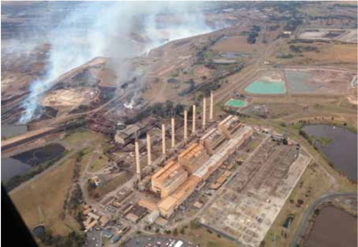
Figure 2.29 Hazelwood mine fire on a 'spike day' – 25 February 2014 116
