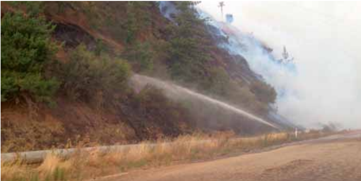
Figure 2.15 Photograph of the northern batters taken in an easterly direction by Mr Shanahan at approximately 4.27 pm on 9 February 2014 71
