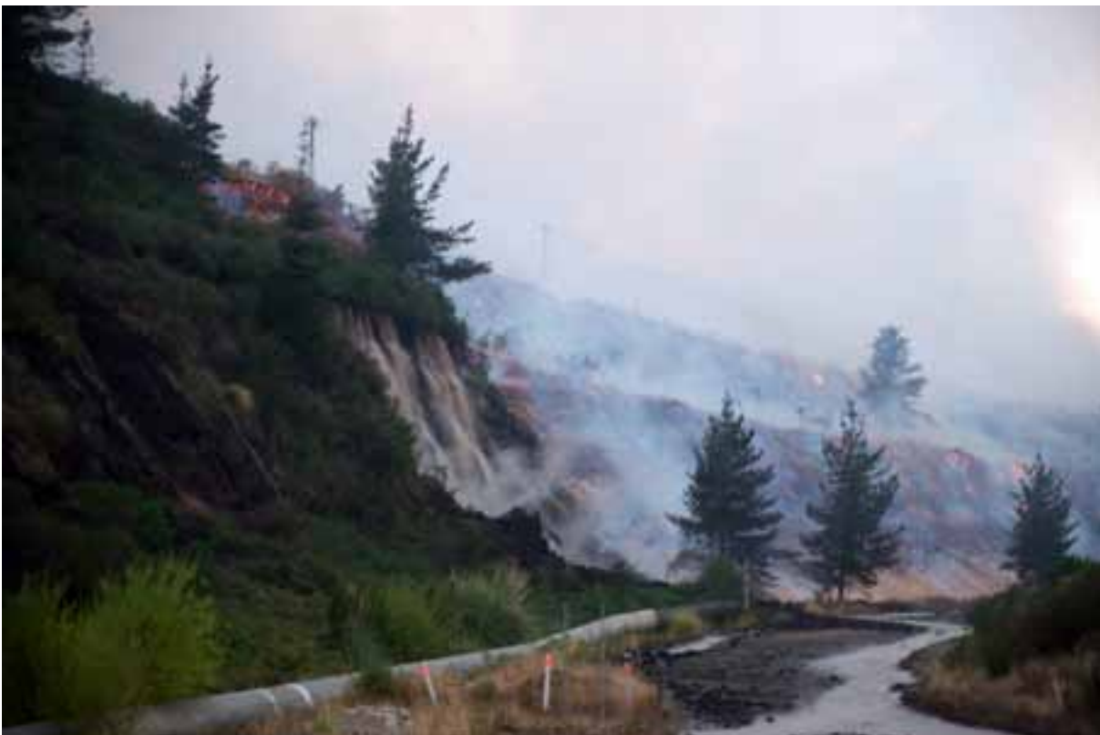
A water-break in the northern batters prevented the fire from spreading west towards the operational area of the mine. Photograph taken by Mr Steley.
