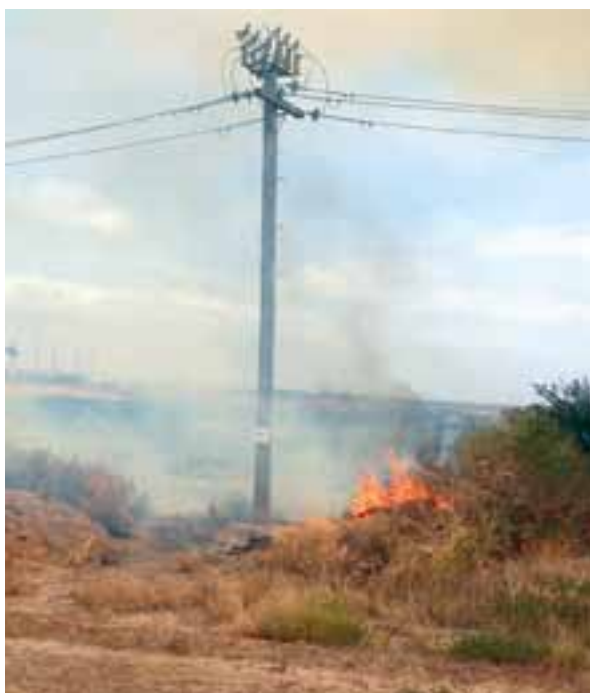
Figure 2.13 Fire burning beneath the power poles in the northern batters at 3.20 pm on 9 February 2014 65
