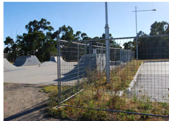
Existing interface between skate park and car park
